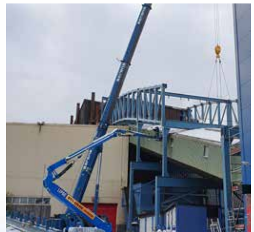
The replacement of a conveyor bridge for raw iron ore transport, LKAB, Sweden
