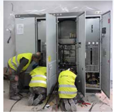
The project providing for the replacement of asynchronous motors together with accompanying equipment, The ELMA-LABIOD cement plant, Algeria
