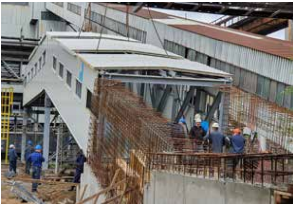
The construction of a conveyor bridge in the Chwałowice coal mine
