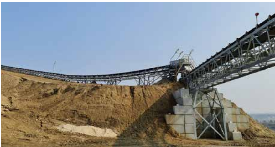
The reconstruction of the post-flotation waste transport system at the tailings ponds in the Bolesław mining and metallurgical complex
