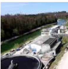
WASTE WATER TREATMENT PLANTS
