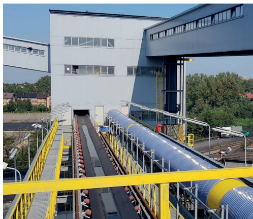
The construction of a stone belt conveying system with a storage bunker and a loading station with a possibility of loading onto trucks in the Janina coal mine
