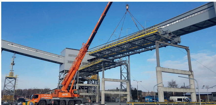
The construction of a stone belt conveying system with a storage bunker and a loading station with a possibility of loading onto trucks in the Janina coal mine
